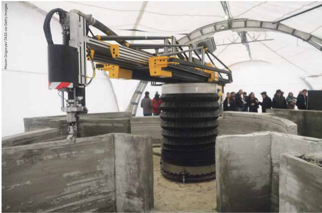
Russian firm Apis Cor is able to print a 400sq-ft concrete house in just 24 hours with no wastage
